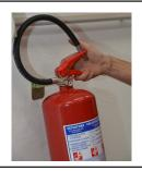
Remove the fire extinguisher from the bracket and check: stability of the bracket, cleaning and general conditions. Check marking label and replace it if damaged.
