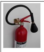
Remove the extinguisher from the bracket and check: stability of the fastening support, cleaning and general conditions.
